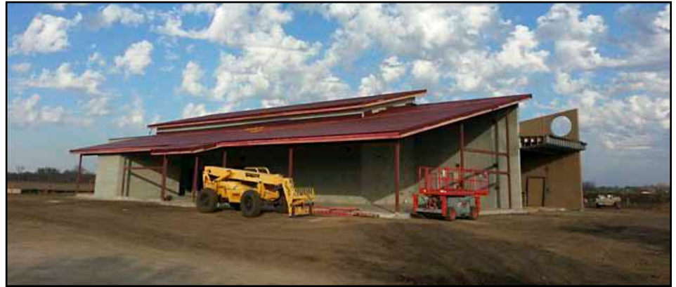
The Clay County Jail project is about four weeks behind schedule, according to Midwest Construction Consultants construction manager John Hansen. An extension is not being granted at this time because Hansen believes the project can be brought up to speed and meet the April 2013 target. (photo: Randy M. Cauthron)
