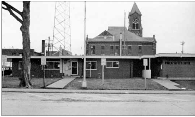
Washington County Public Safety Center
